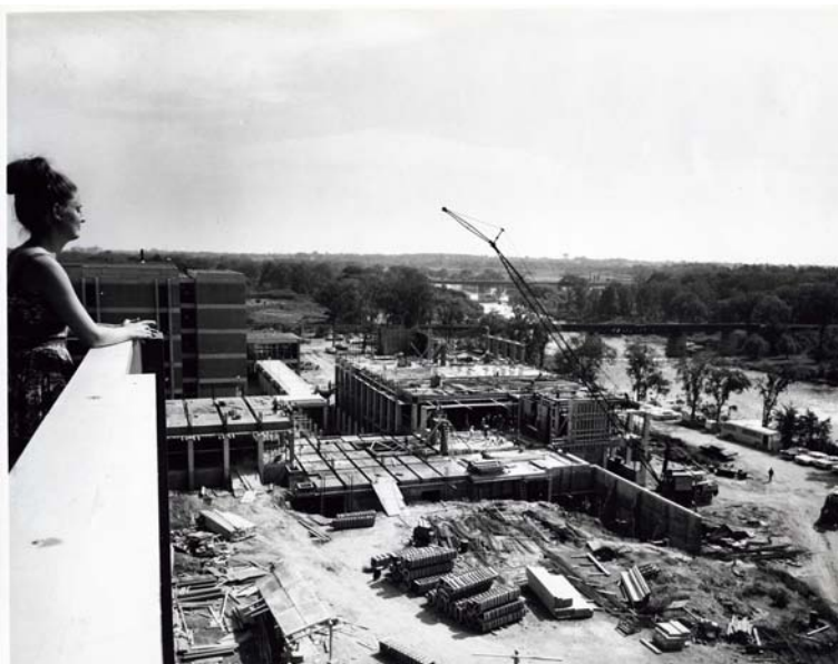
Carleton University Under Construction Carleton University Archives and Research Collections
