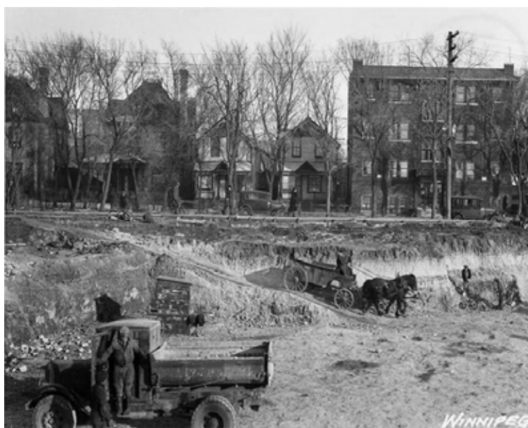
Archives of Manitoba, Winnipeg Buildings, Municipal, Civic Auditorium 9. Construction of the Civic Auditorium, 1932.
