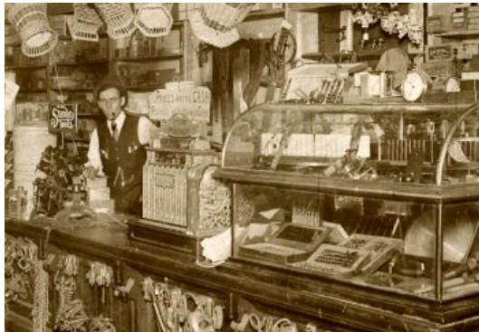
Interior of Sackville and Sons Hardware, Riversdale, ca. 1911-14. City directory listing advertised "Hardware, Stoves and Harness. Harness repairing a speciality." Saskatoon Public Library Local History Room, photograph LH-1919.
