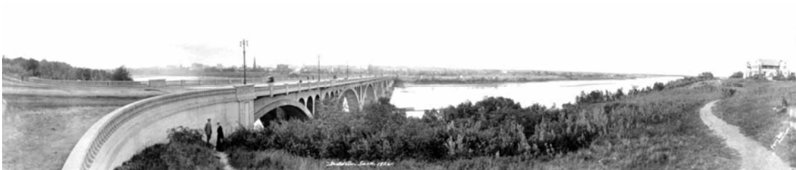
Newly completed University Bridge; South Saskatchewan River in background, University of Saskatchewan President's Residence at far right. Photograph by Gibson, 1926. University of Saskatchewan Archives, Photograph Collection, B-266.
